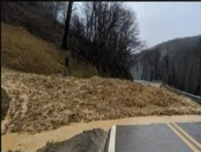
Canyon Roads Blocked by Mud & Rocks
